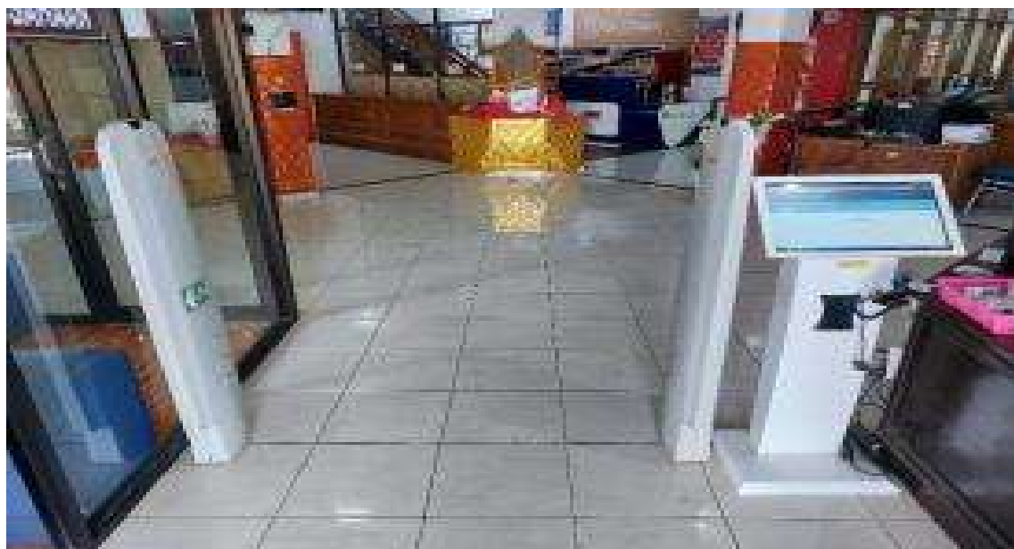
Pintu Detektor/Auto Gate, Tripod Vertical Turstile barrier Gate
